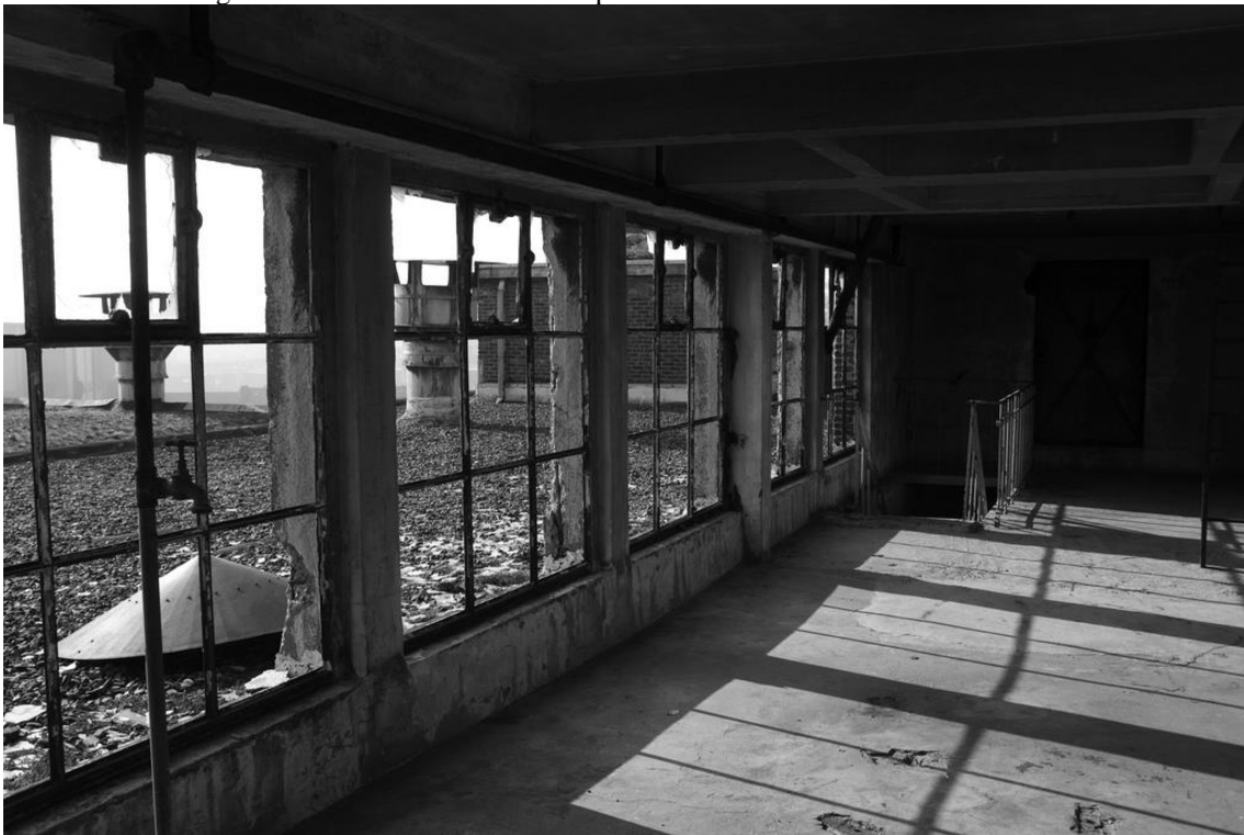
Figure 2: Interior view before adaptive reuse (currently meeting room). Source: Bart Plessers.
