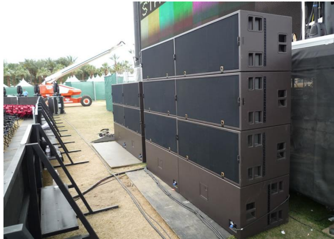
Figure 15 : Cardioid setup for subwoofers (L-ACOUSTICS SB28).
